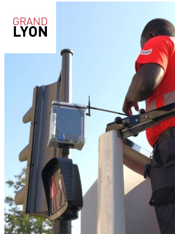
Deployment in Lyon: 12 sensor nodes + 1 gateway
